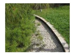
Bioswales are stormwater conveyance systems designed to remove silt and pollutants from surface runoff water. They consist of a swaled drainage course with gently sloped sides and filled with vegetation, compost and/or riprap. The path where the water flows, along with the wide and shallow ditch, is designed to maximize the time water spends in the swale, which aids in the trapping of pollutants and silt.
