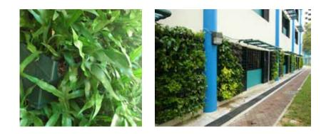
Prince's Hi-Green Vertical Wall Systems use a specialised "live" hydroculture technique to ensure sustained plant health. System components include Prince's unique water and nutrient-absorbent planting medium, Hi-Green Lite Composite, together with the irrigation system and, where necessary, water reservoirs in individual planters. These components reduce the watering requirement and helping to make Hi-Green Vertical Walls ultra-low maintenance systems.
