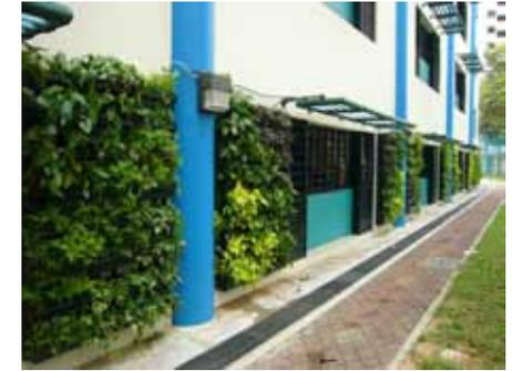
Prince's Hi-Green Vertical Wall Systems use a specialised "live" hydroculture technique to ensure sustained plant health. System components include Prince's unique water and nutrient-absorbent planting medium, Hi-Green Lite Composite, together with the irrigation system and, where necessary, water reservoirs in individual planters. These components reduce the watering requirement and helping to make Hi-Green Vertical Walls ultra-low maintenance systems.
